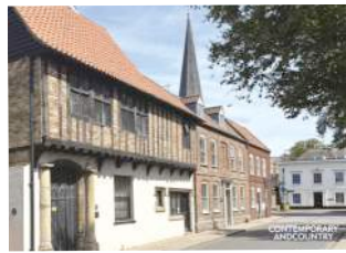
Woolmarket House, the home of Contemporary and Country and new exhibition space The Viewing Room
