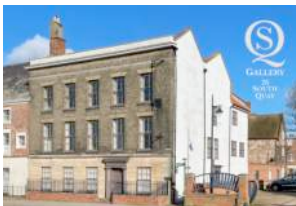
The recently renovated South Quay Art Gallery & Learning Centre, South Quay, Great Yarmouth Photo Pete Huggins
